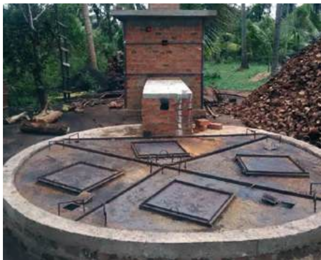
Haritha Angara Environment friendly closed charcoaling pit
